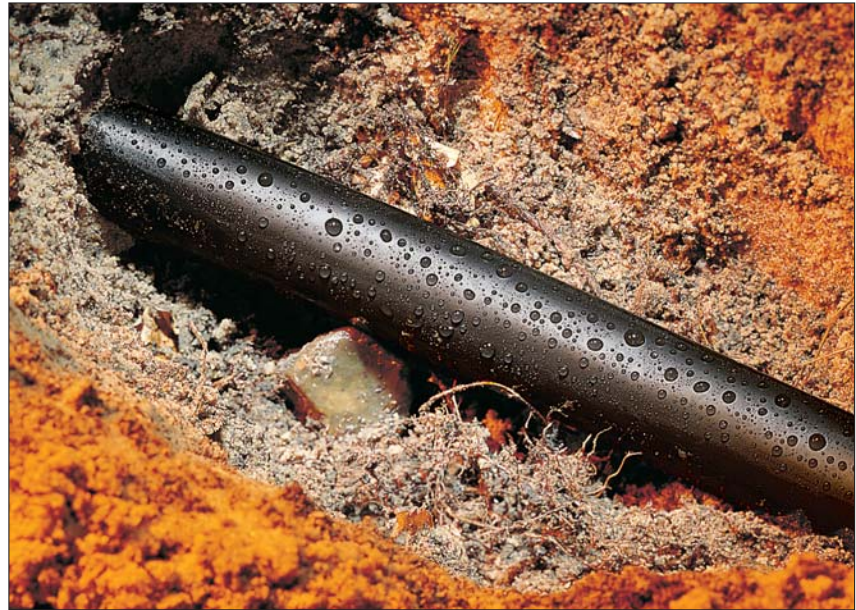
TREDUX HA47 - application below ground.
